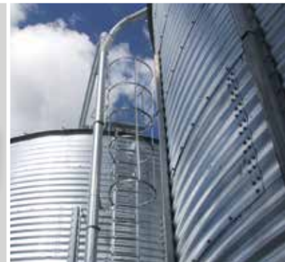
Pipe line for filling outdoor steel silos.
